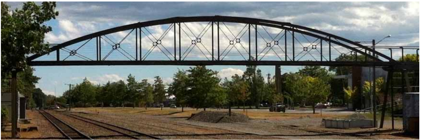
New Zealand's first Blue Plaque commemorating the Ashburton Railway Footbridge was unveiled in November 2017.
