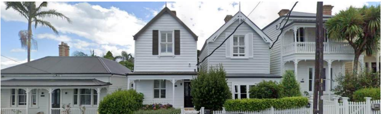
Villa (left) with cottages (centre and right) in Ponsonby. Google Street View looking north from Cowan St. Photo / Auckland's Special Character Areas Report.
